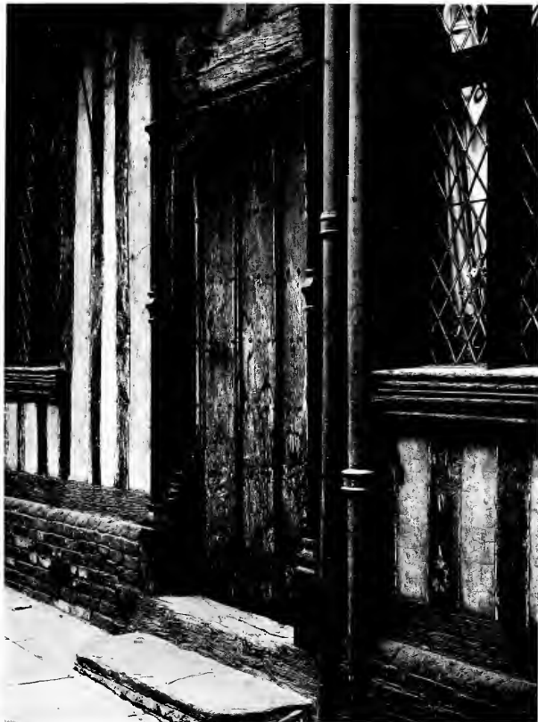
OLD OAK HOUSE, SIDE ENTRANCE DOOR
